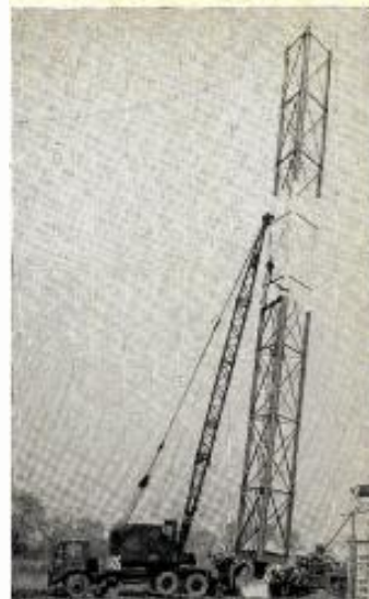
FIRST 80 feet of WLWC (TV) Columbus' 578 foot tower, designed and fabricated by International Derrick & Equipment Co., is hoisted into place. The Crosley Broadcasting Corp. station is assigned Channel 3 and expects to start operation by March 27.
